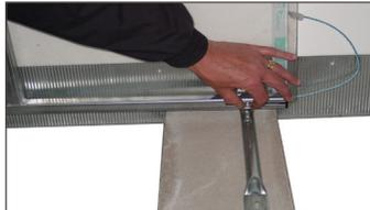
2. Position the cover over the window well opening to determine placement of the side tube mounts for each side. Remove the cover to mount the side tubes in holes provided\*. Position and install the front tube mount on the "face" of the areawall. Use multi-purpose exterior grade screws. For concrete areawalls, pre-drilling screw holes will be required.
