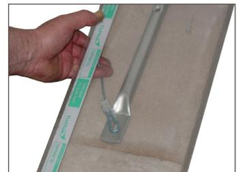
4. Attach the safety retainer-hinge lanyards via the front screw holes in the side tube mounts. \*Alternatively, anchor the loop end of the lanyard to the home foundation or directly to the areawall itself depending on your particular application. Allow for enough lanyard length to allow the cover to pivot up and stay propped open against the side of the house for window well access.
