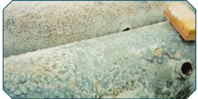
Figure 9: Heavy wet storage stain
