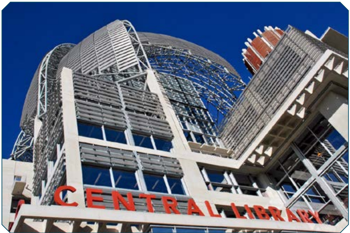
San Diego Central Library utilizes galvanized steel
